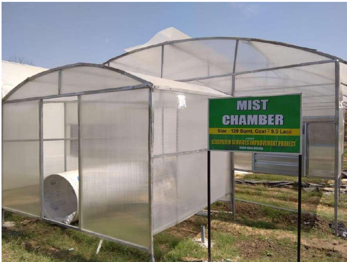
Figure 5 Construction of Mist Chamber
