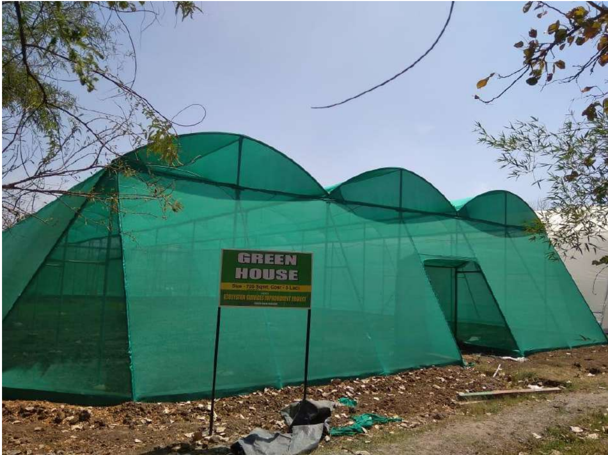
Figure 1 Constructed Green House
